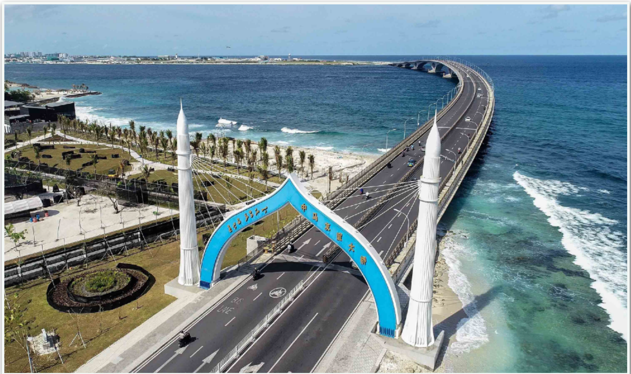
Finished in 2018, the China-Maldives Friendship Bridge stands as the hallmark initiative of China's infrastructure surge in the Maldives.
